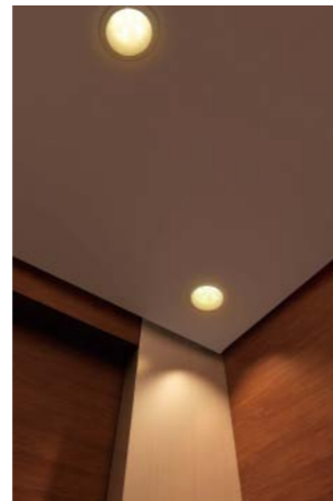
Ceiling: Painted steel sheet (Y033) Lighting: Downlights (LEDs)
